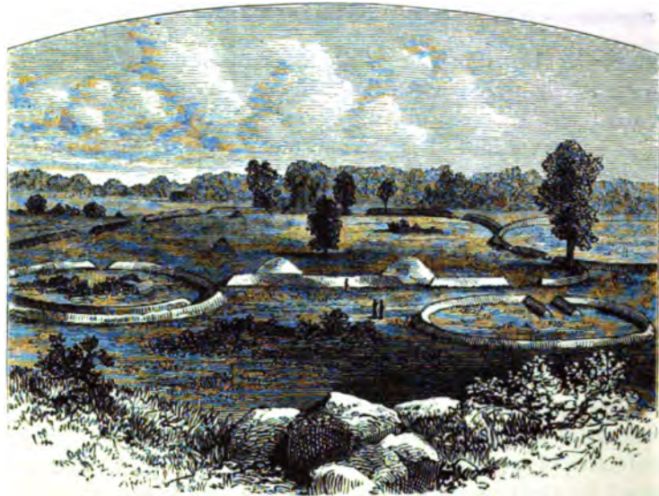
Earthworks in Ohio.
